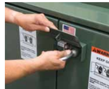
Switch-Handle Operation - handle unfolds and clip slides over joint to fix handle in extended position
