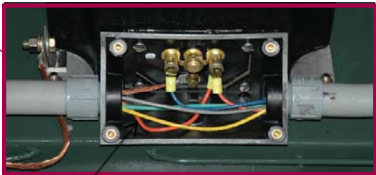
Concealed Color-coded control wire.
